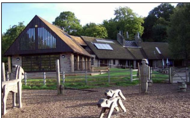
Beechenhurst before the new extension
